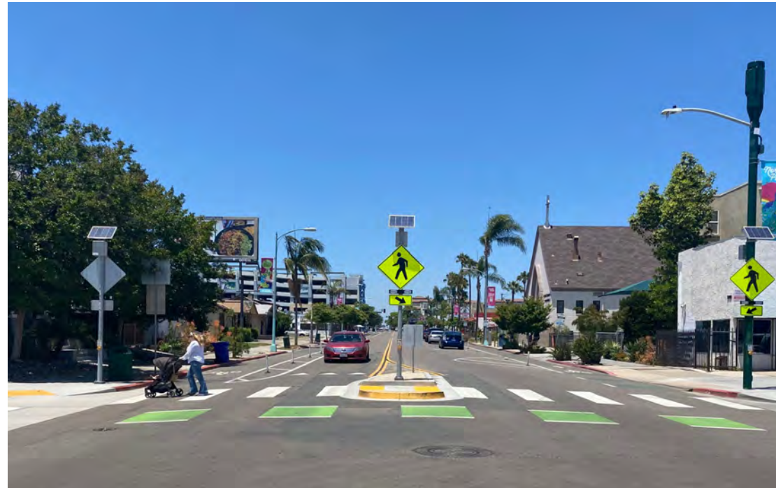
Enhanced pedestrian treatments at 30th Street and Landis Street in North Park
