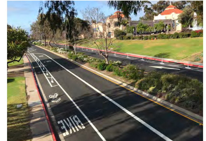
Road resurfacing with multimodal facilities on Park Blvd Source: City of San Diego
