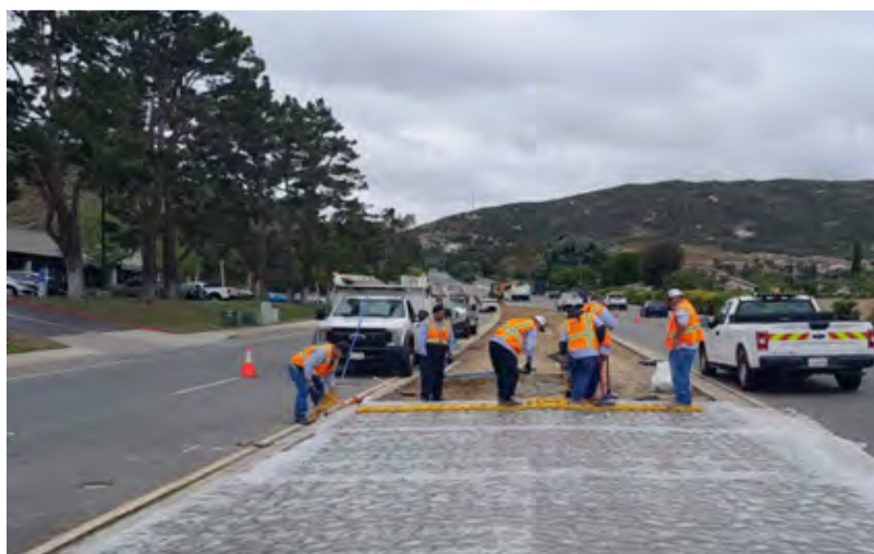
City crews constructing a center median.
