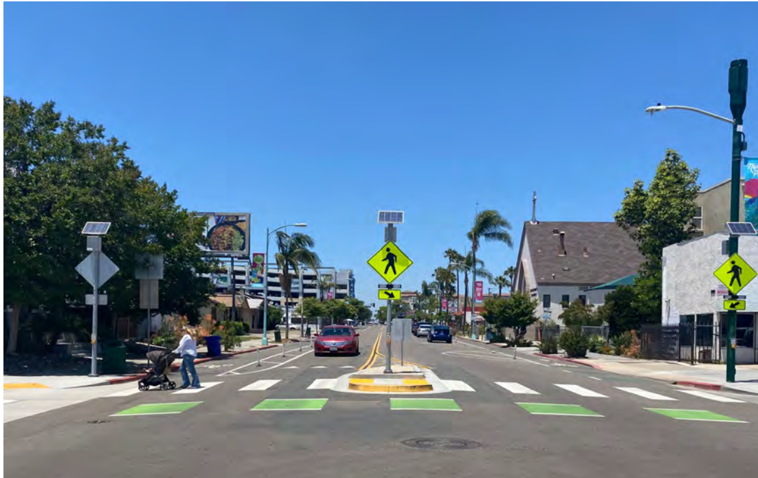
Enhanced pedestrian treatments at 30th Street and Landis Street in North Park
