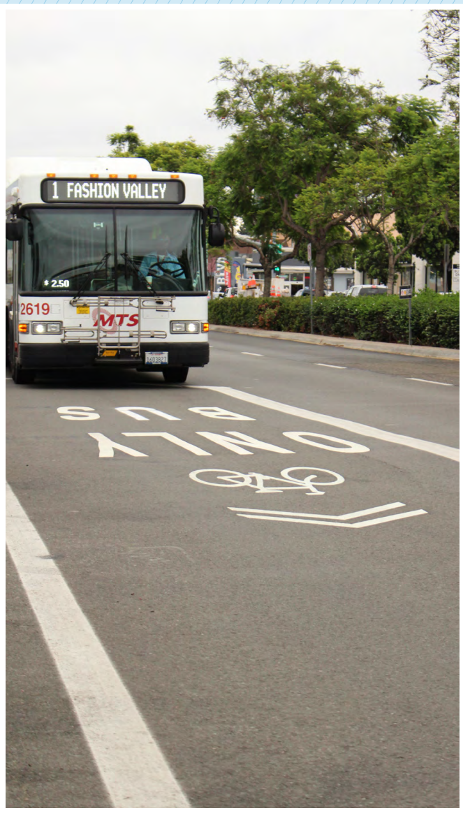
Flexible (flex) lane along El Cajon Boulevard
