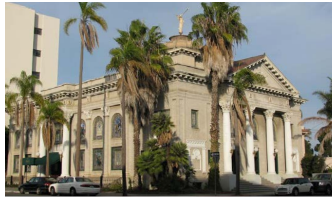
The Park Place Methodist Episcopal Church is a remarkable example of Classical Revival architecture in the Bankers Hill/Park West neighborhood.
