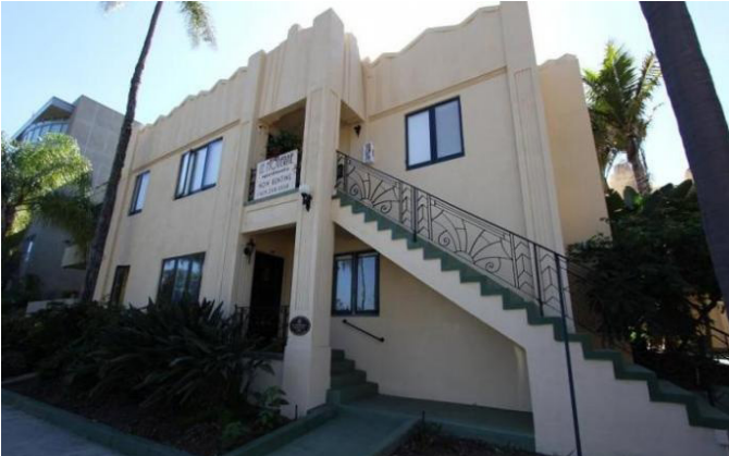
Le Moderne Apartments, built in 1930, is an early and excellent example of the art deco architecture in style during the 1930's and 1940's.
