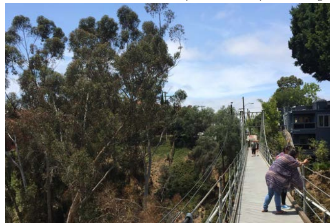
Spruce Street Suspension Bridge
