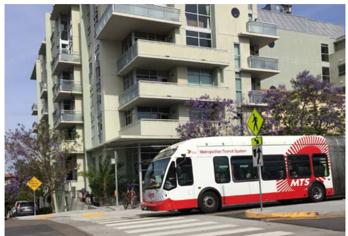
Encouraging mixed use development along commercial corridors, served by transit is a major focus of the Community Plan.
