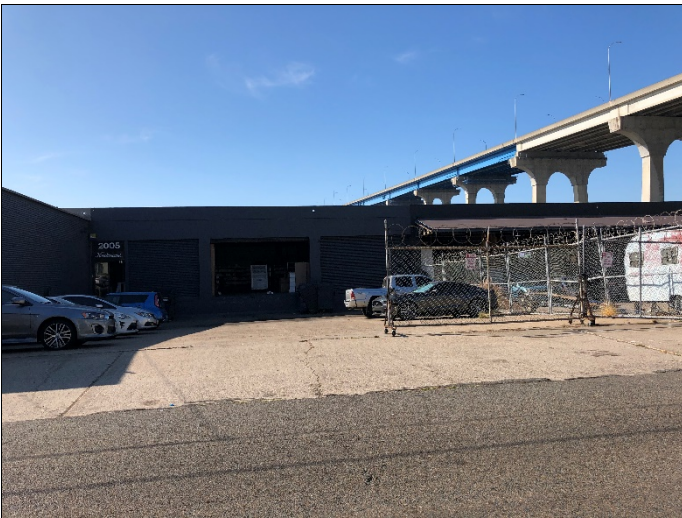
33. Representative view of southwest-adjacent EQ Studios (2001-2009 Main Street)
