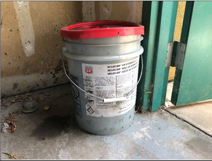
7. View of open container of hydraulic fluid stored in elevator equipment room and surficial spill
