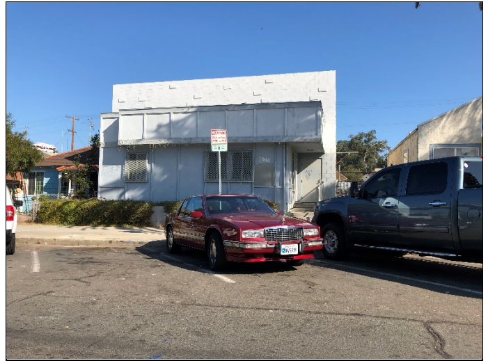
28. View of northeast-adjacent warehouse (2046 Newton Avenue)
