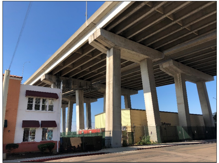
26. View of northwest-adjacent Caltrans Coronado Bridge staging facility (1995 Newton Avenue)
