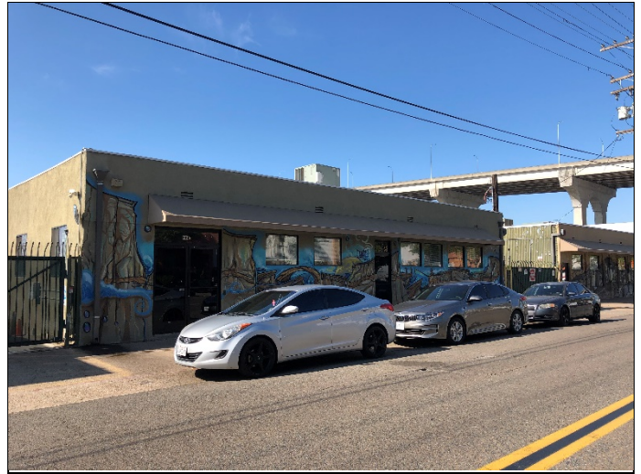
32. View of southwest-adjacent light-industrial facilities (2011-2049 Main Street)
