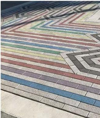
Example of a pattern treatment type: colored concrete pavers
