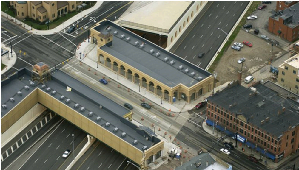
Photo showing the completed version of The Cap at Union Station
