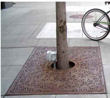
Tree grates should be used in commercial and mixed-use areas to reflect street and neighborhood character and protect trees.
