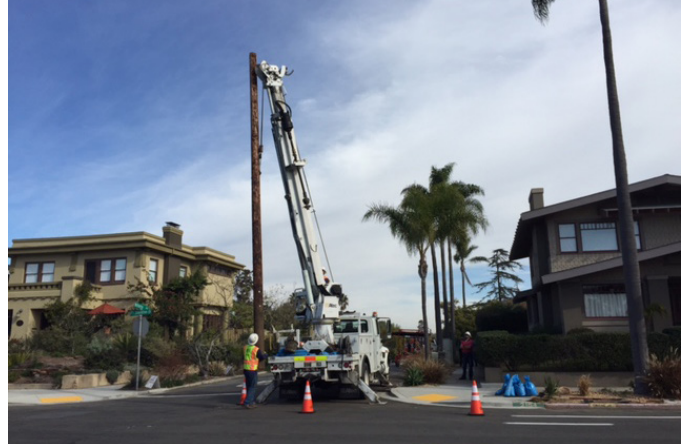
The City of San Diego works in collaboration with local utility providers to underground overhead utility lines with safer, more reliable underground utility systems.
