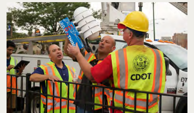
Installing AoT sensors, Chicago Source: University of Chicago, 2016
