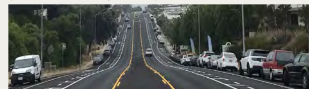
Road resurfacing with bikeway on Gramercy Drive Source: City of San Diego
