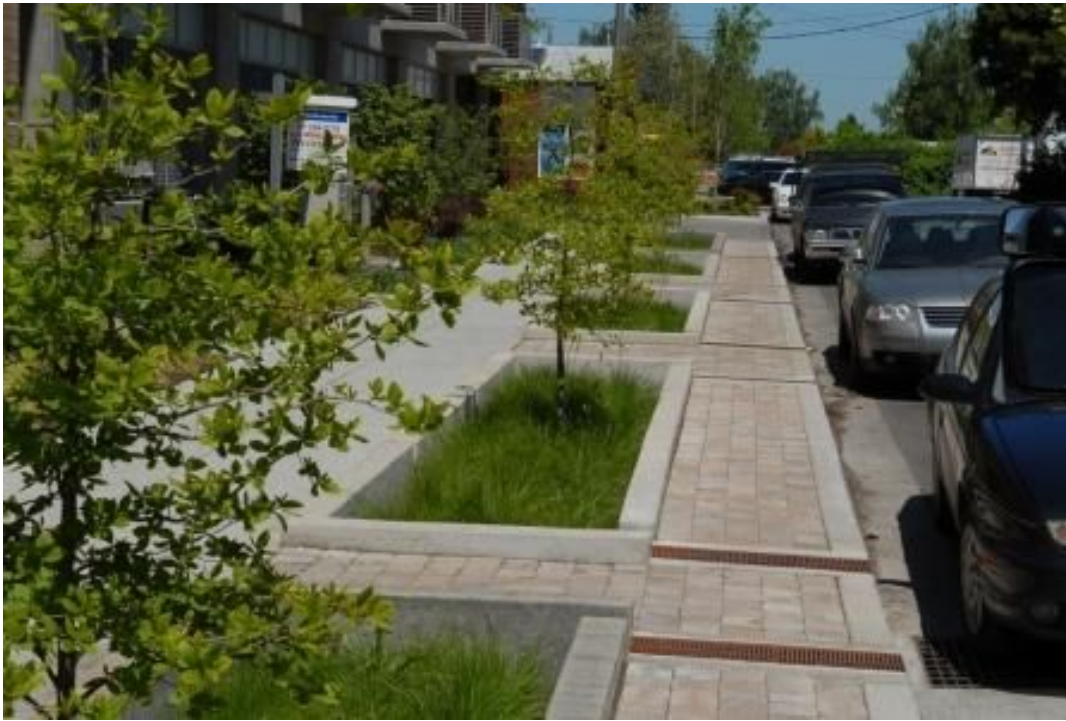
Flow-through stormwater planter
