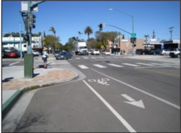
Curb Extension / Bulb-outs
