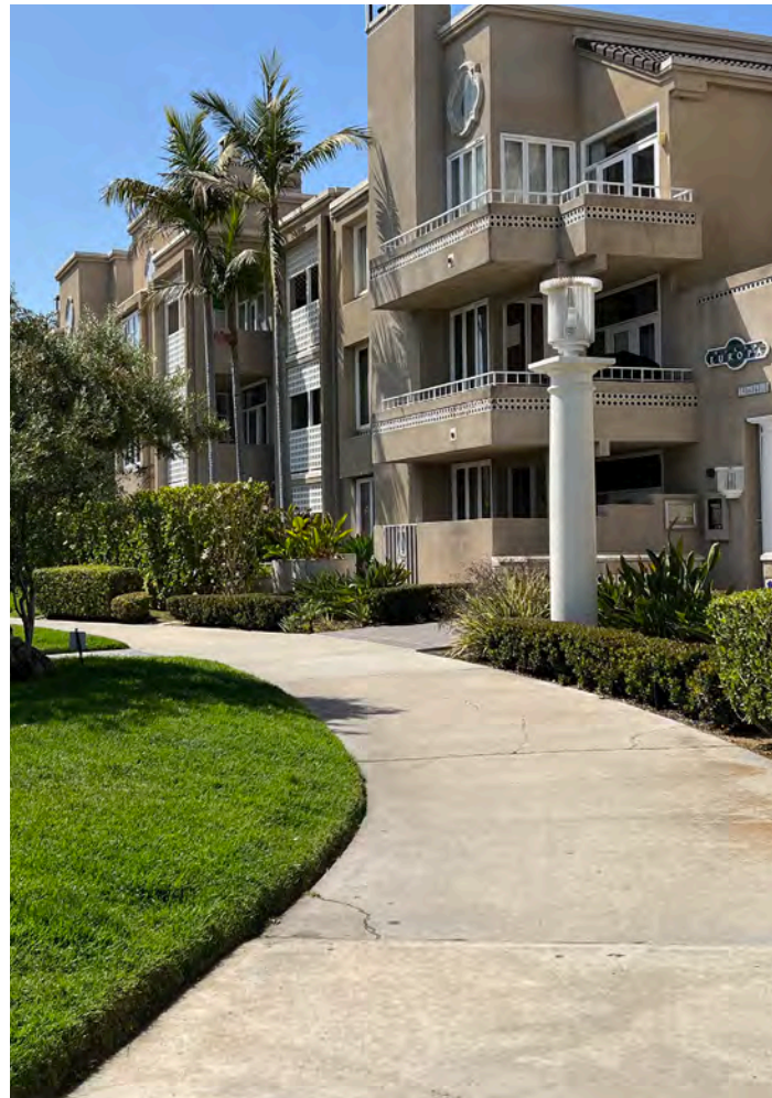
Accessible, interconnected pedestrian routes improve walkability.
