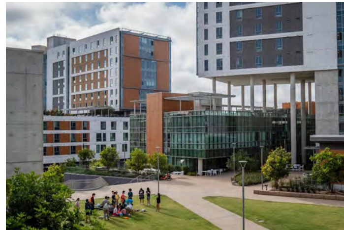
Once a parking lot, the North Torey Pines Living and Learning Neighborhood is now a mixed-use community on the UC San Diego campus that encourages social and academic interactions at multiple scales.
