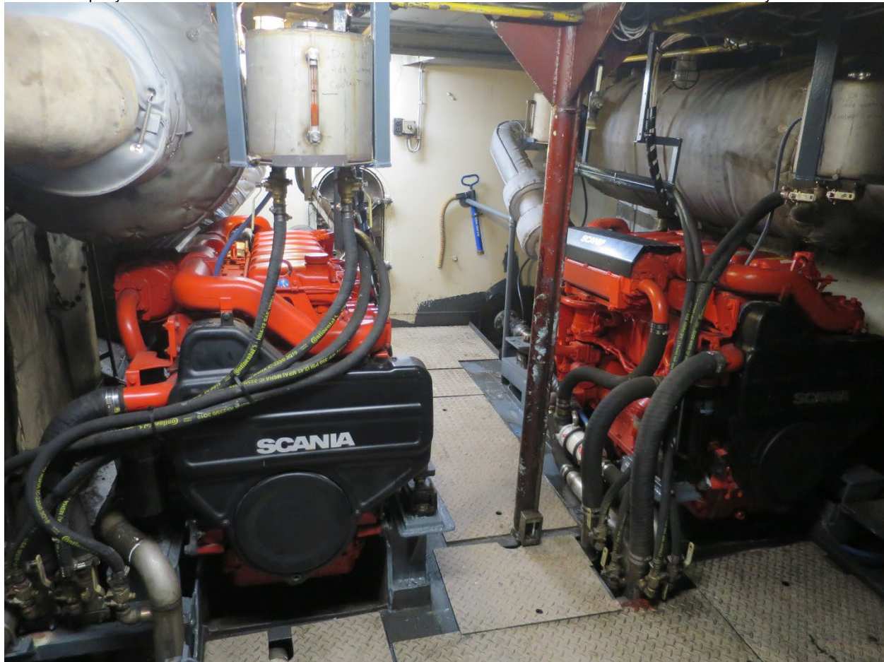
Photo 18. Cabrillo , below deck, engines and bulkhead walls
