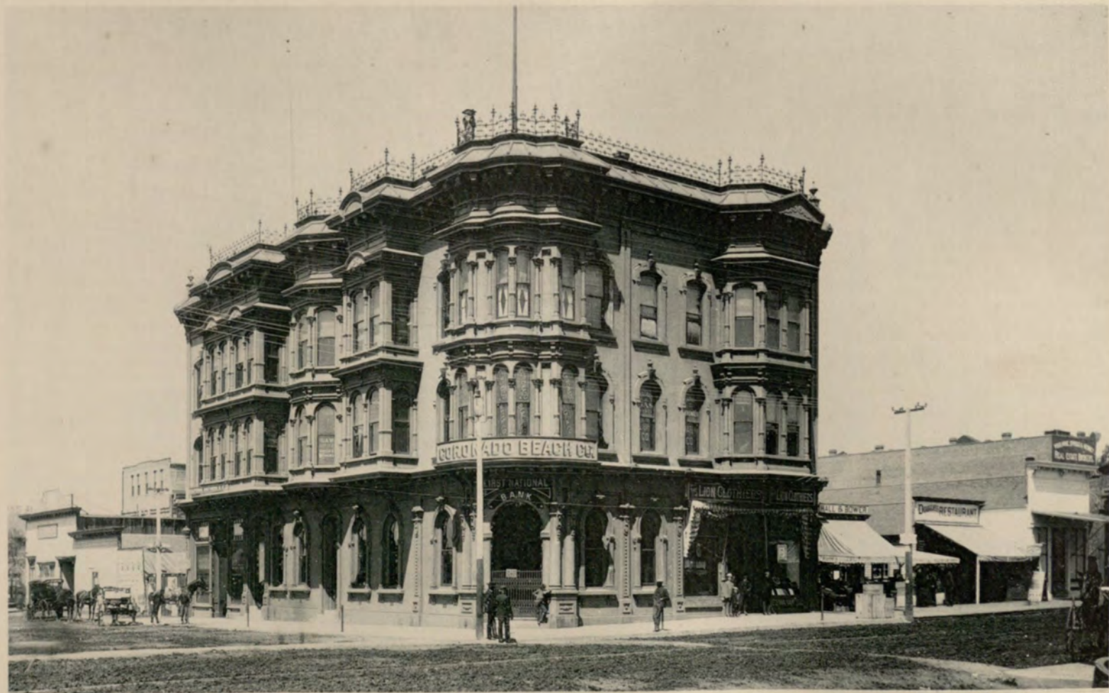
First National Bank, corner Fifth and E streets.
