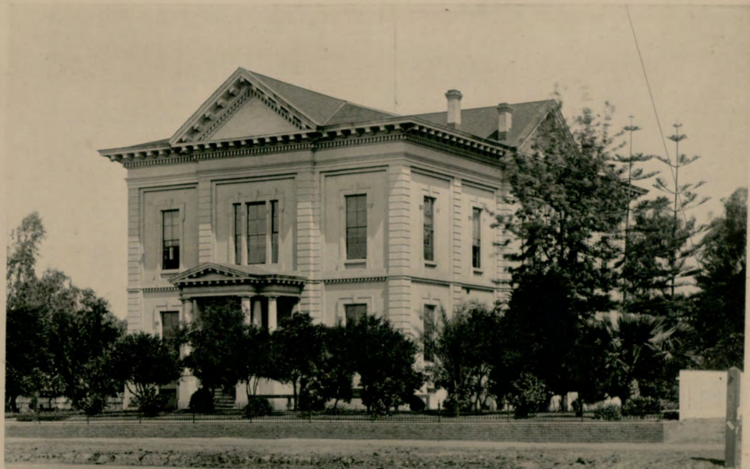
County Court House, San Diego.
