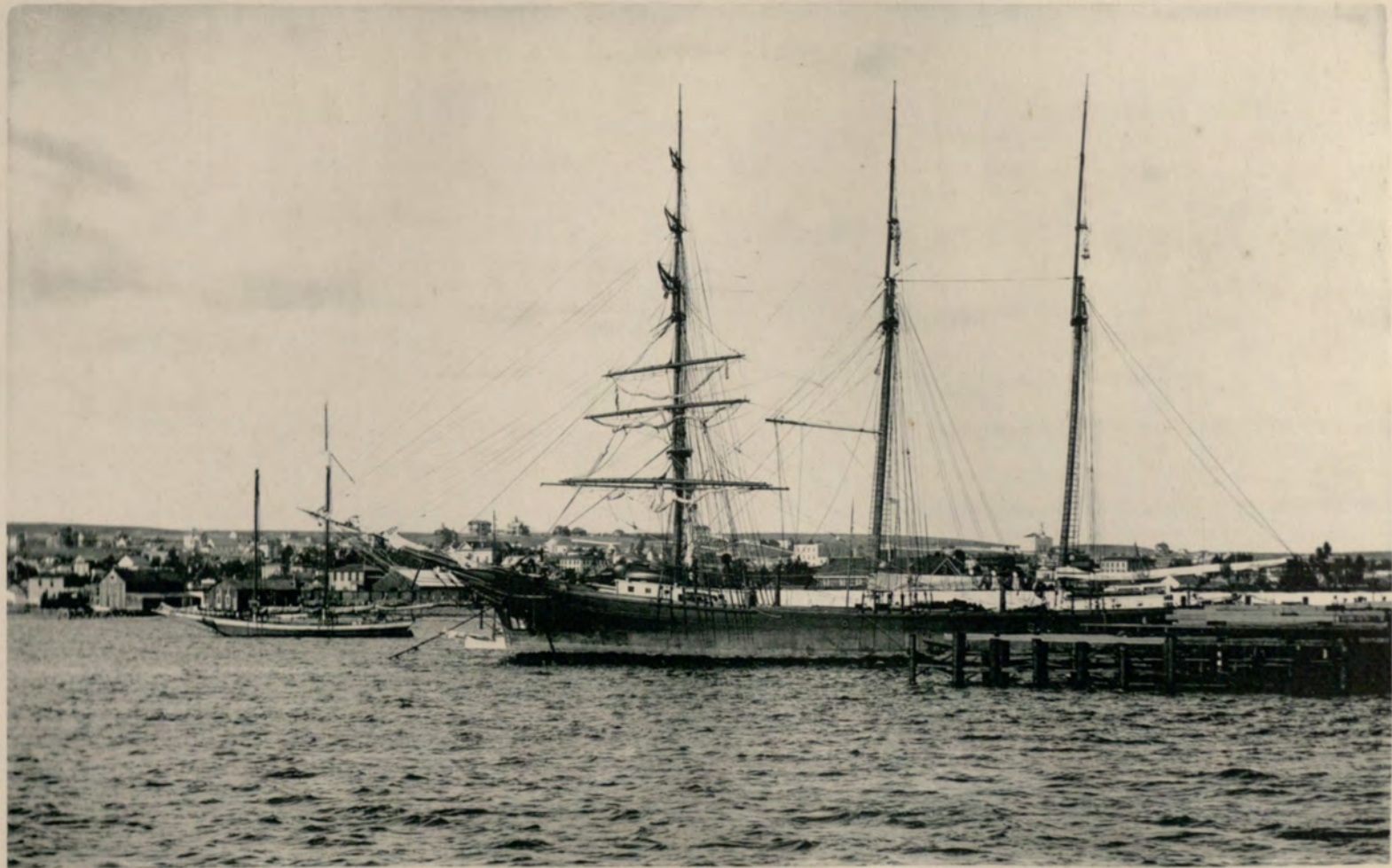
City Water Front—Babcock & Story Wharves.
