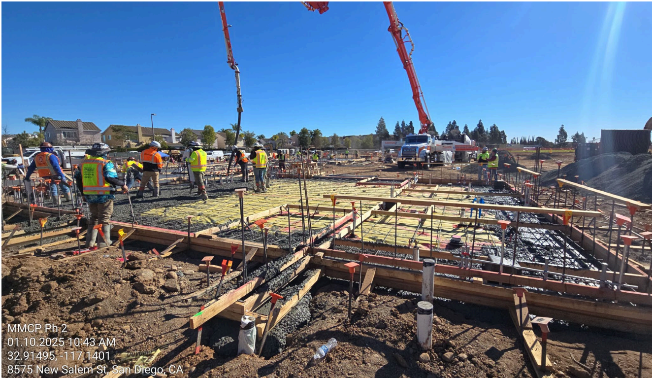
Aquatic building slab and footings.
