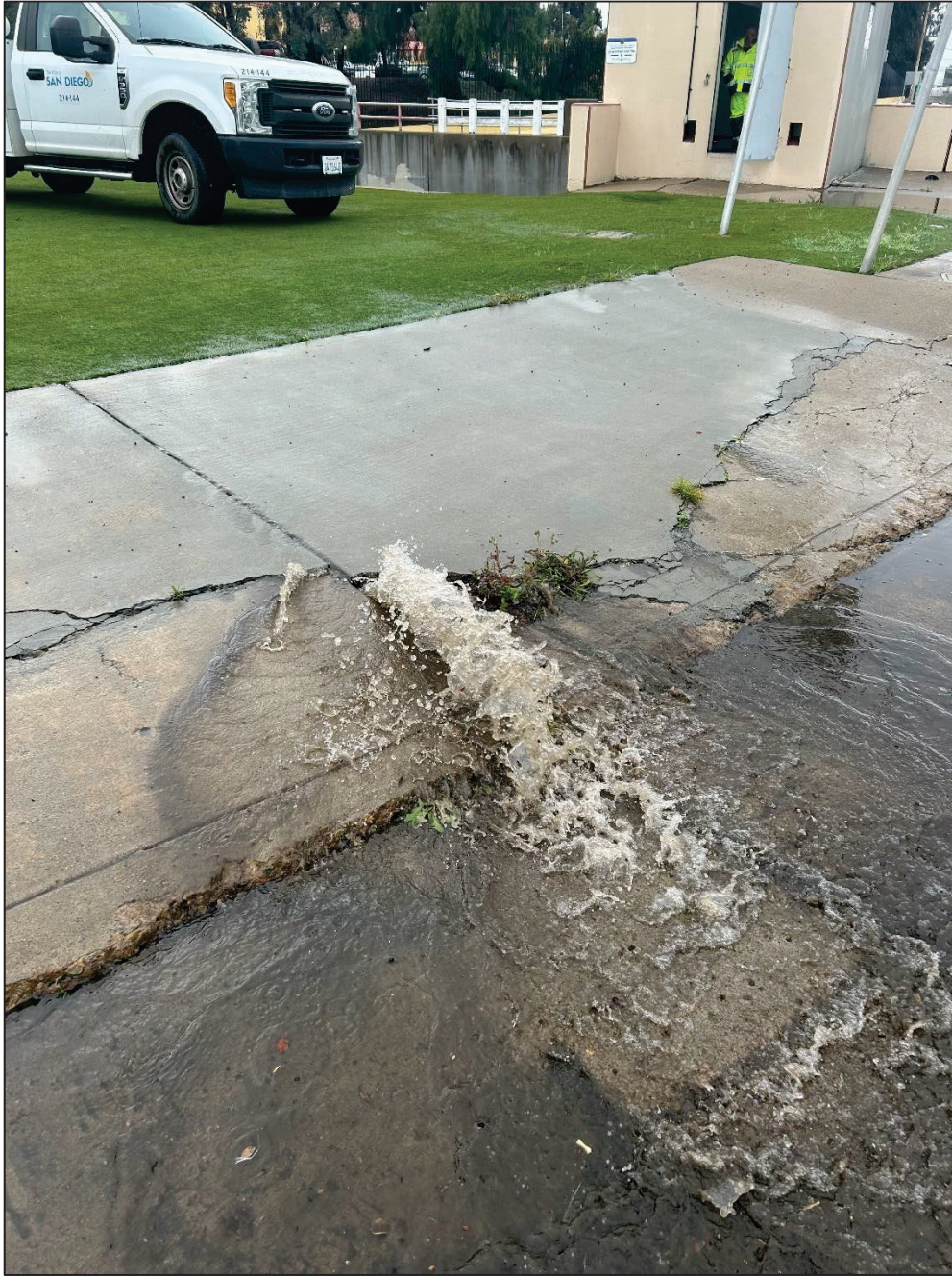
Jan 22, 2024 – Stormwater discharging through driveway on SB Pacific Highway during a rain event.
