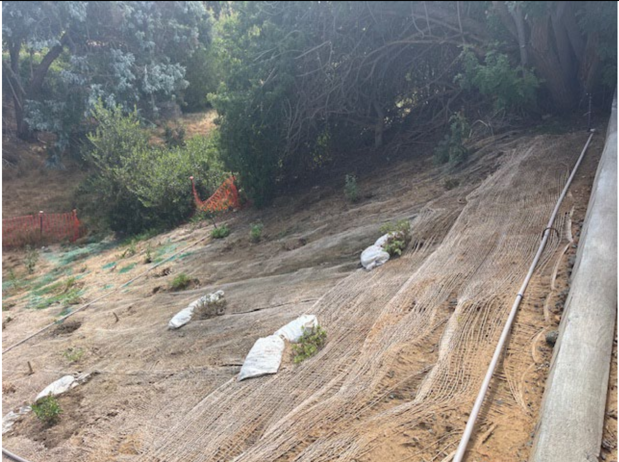
Photo 3. Overview of the site. View southeast.
