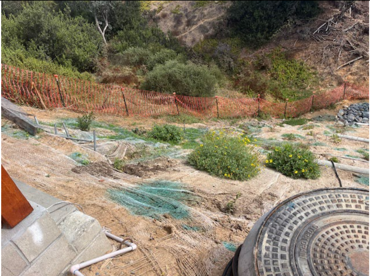
Photo 2. Overview of the site. View northeast.
