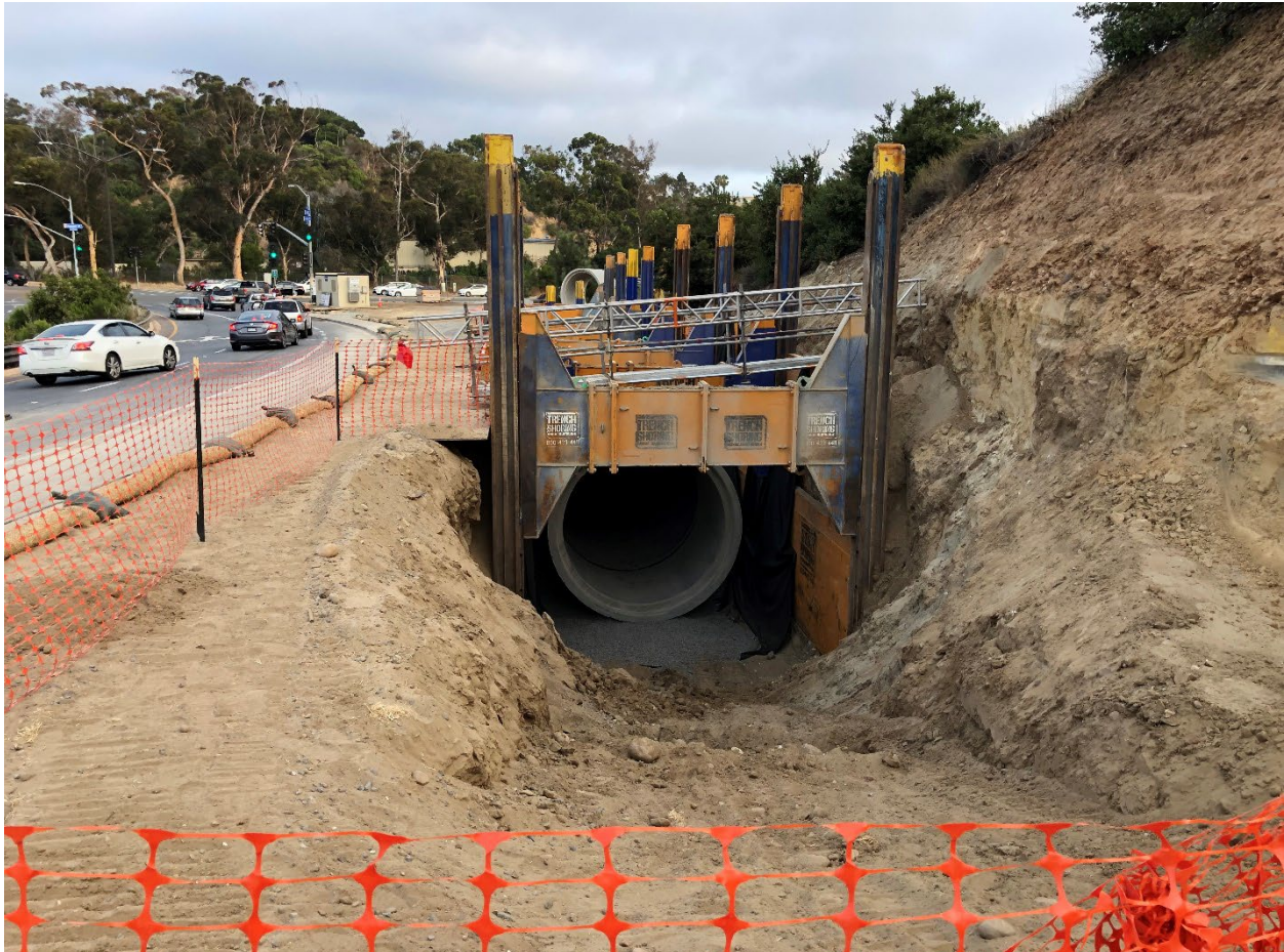
Nasland Project – City of San Diego Florida Drive Emergency Storm Drain
