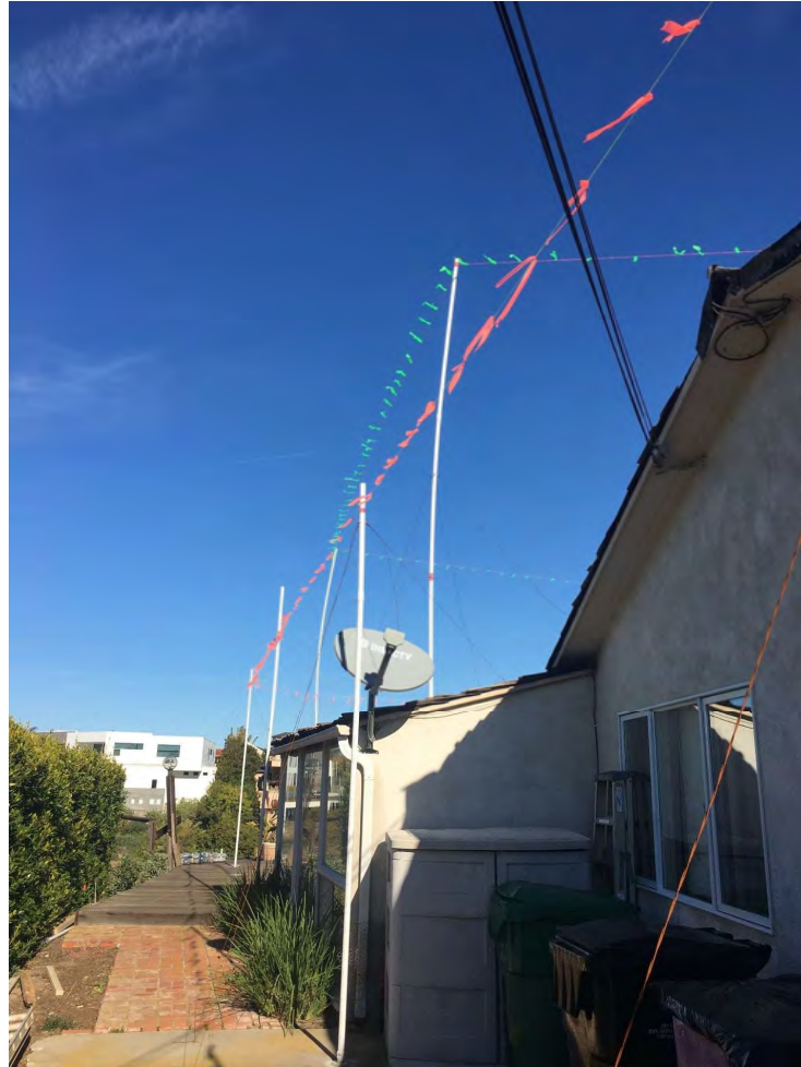
West Lot Line View
