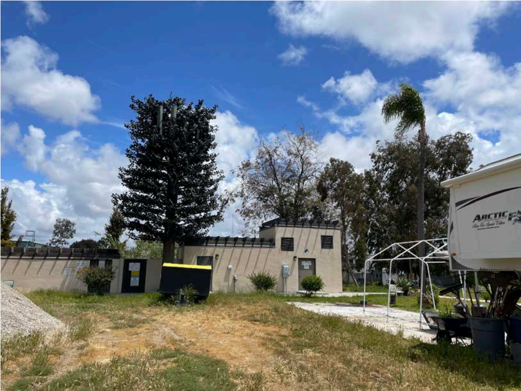
West Elevation (Photo 1)
