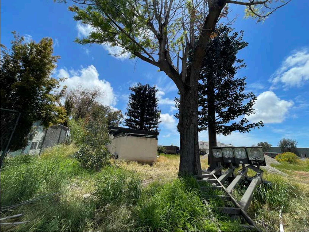
North Elevation (Photo 2)
