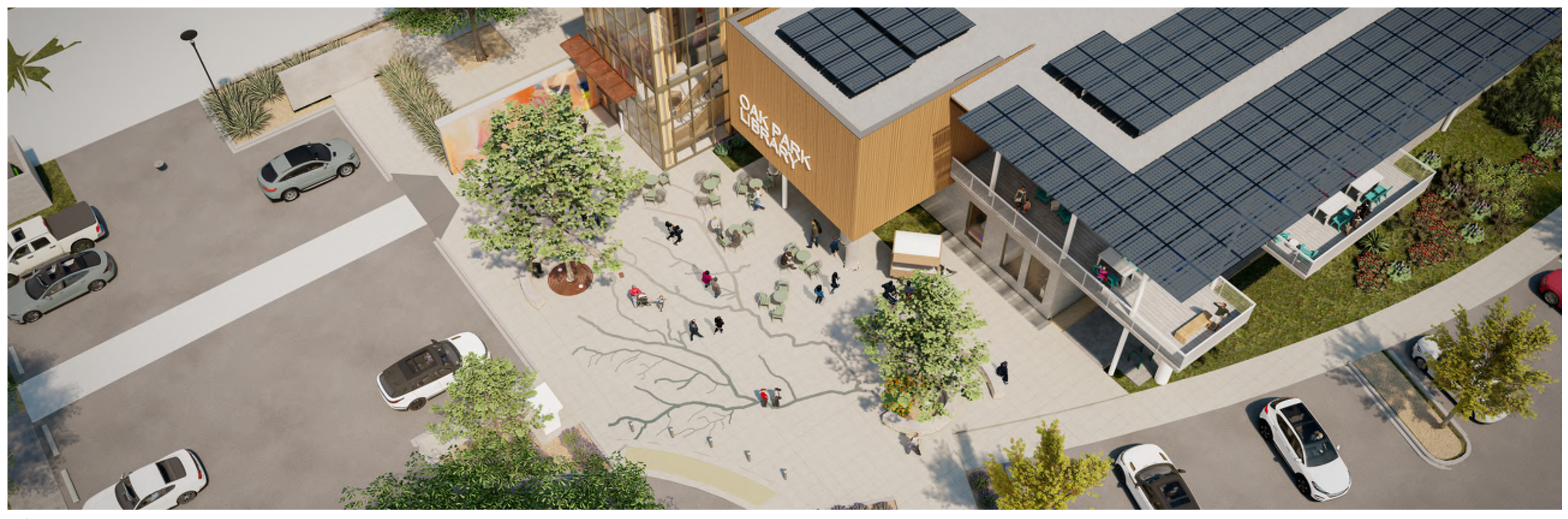
2 Recessed into the Plaza, an aerial view of Chollas Creek watershed is etched into the concrete symbolizing unity with the park.
