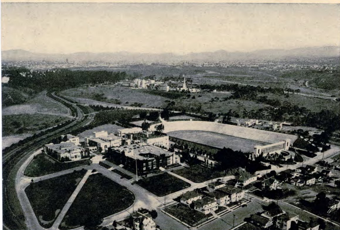
Aerial view of the third largest city park in America. The San Diego High School and Stadium occupies the foreground. In the middle distance is to be seen the great 1,000-bed U.S. Naval Base Hospital, a unit of 25 buildings, costing $5,000,000
