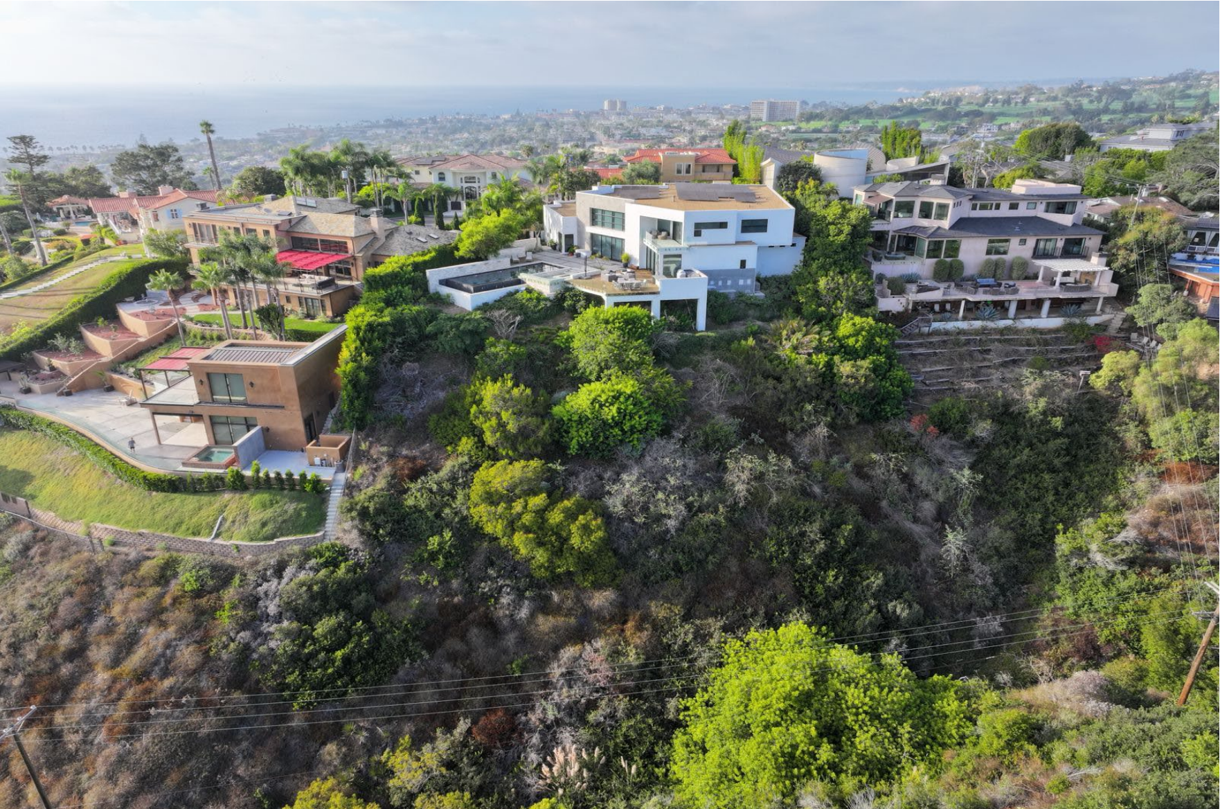
AERIAL VIEW OF THE HOMES ACROSS THE SMALL FINGER CANYON FROM THE GARCIA HOME. THESE HOMES ARE DETAILED ON SLIDES 28, 29 AND 30
