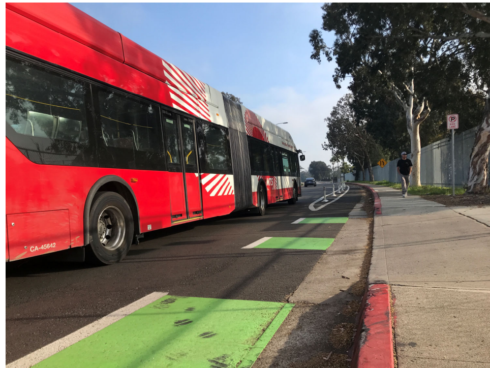
FIGURE 5-20 BICYCLE FACILITIES AT DRIVEWAYS
