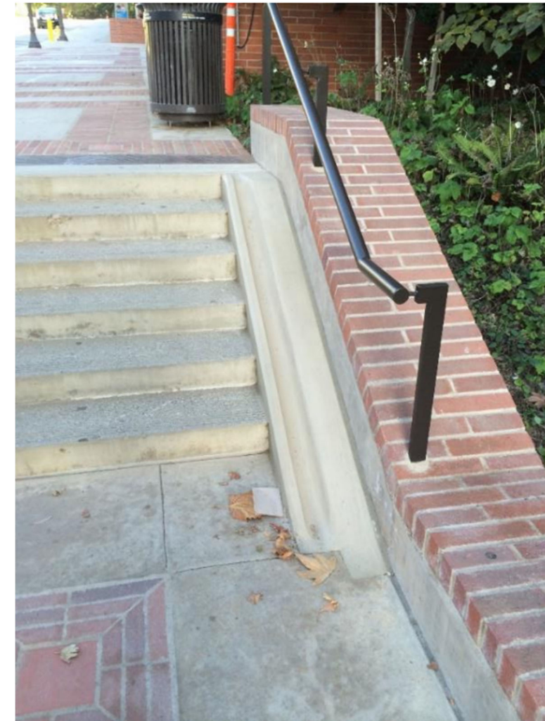
FIGURE 3-33 BICYCLE ACCESS CHANNEL
