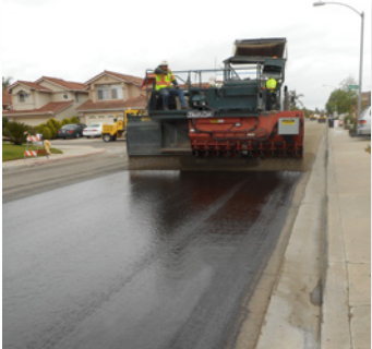
Slurry seal is applied after the crushed rock layer has cured for 3 days
