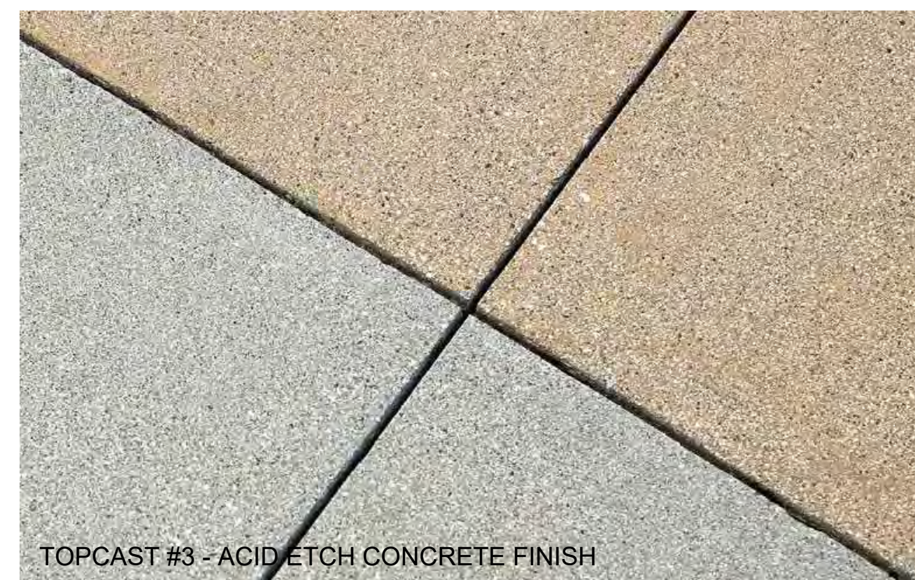
TOPCAST #3 - ACID ETCH CONCRETE FINISH
