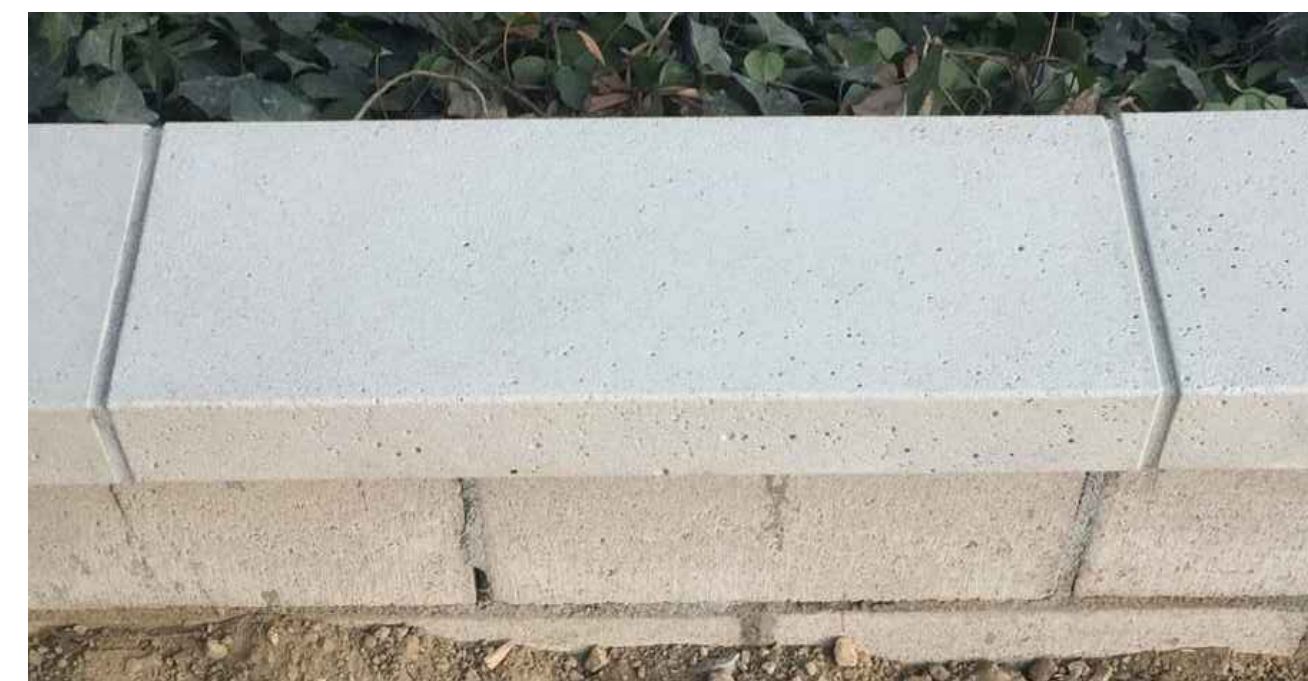
SMOOTH CONCRETE WALL CAP
