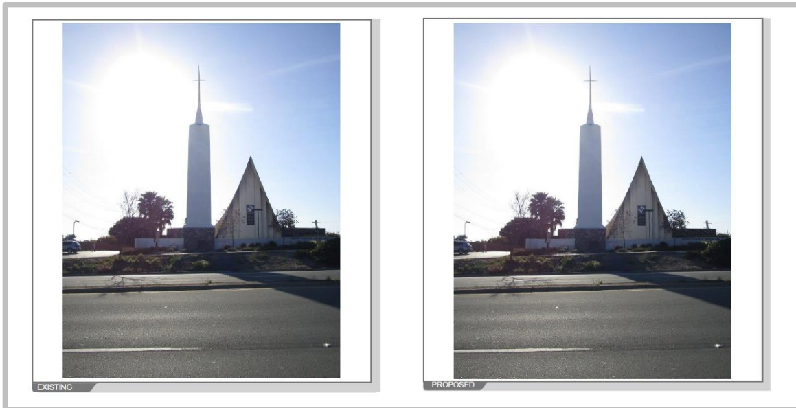
Figure 2 Steeple Conceals Antennas
