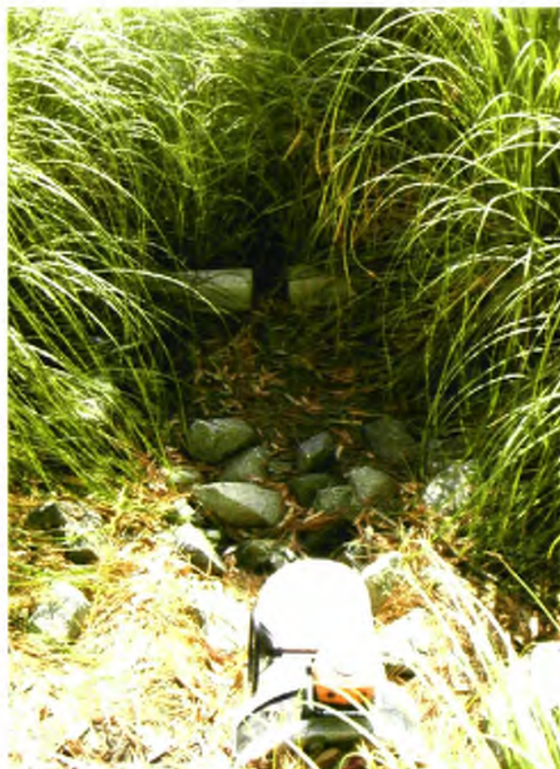
2) View of south storm water outfall looking east.
