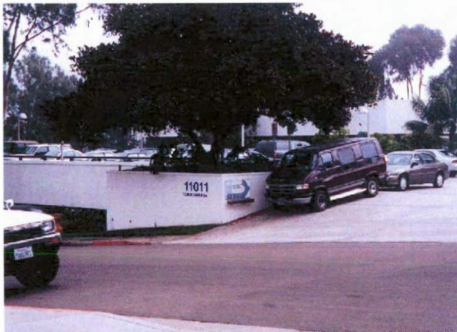
Photo 2 – Discharge point with shutoff valve at the southeast corner of the facility
