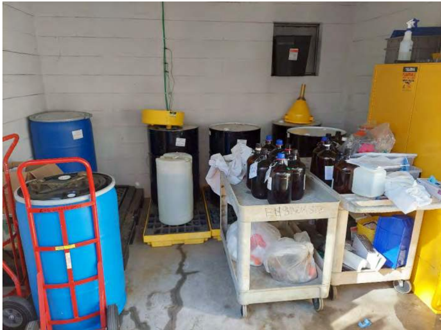
Photograph 22: View of the hazardous waste storage area at the separate utility building.
