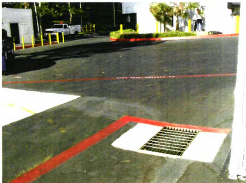
2) View of south delivery area storm drain inlet looking west.
