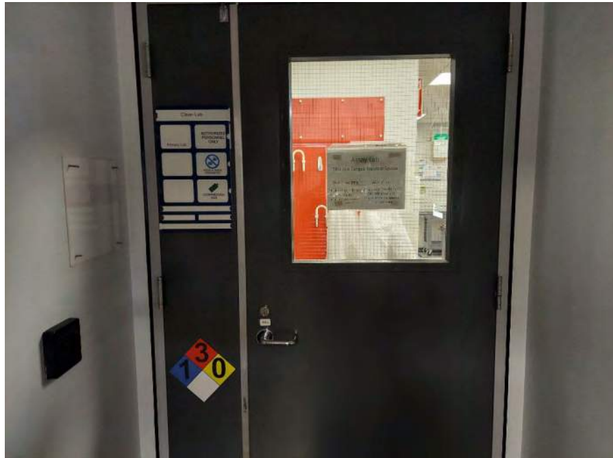
Photograph 7: View of entrance to the clean lab on the second floor. Access was not granted to enter this space.
