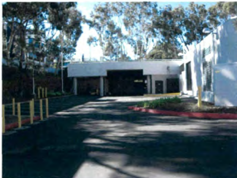
Photo 2: View towards the south of the covered parking structure along the west side of the facility.
