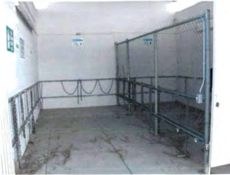
Photo 3: View of interior of chemical storage building.
