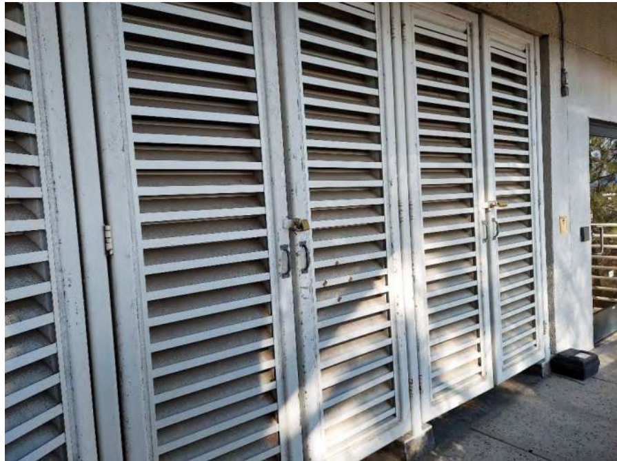
Photograph 19: View of materials supply closet along the southwest exterior wall of the main building.
