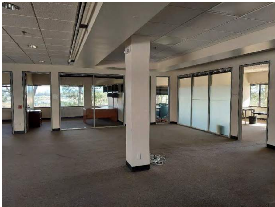
Photograph 6: View of empty offices on the second floor.
