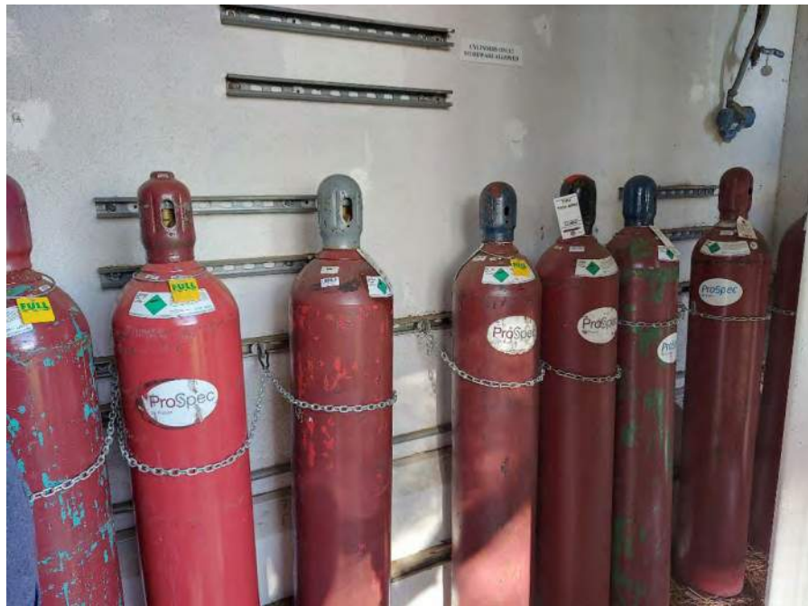
Photograph 20: View of eight 304 cubic-foot compressed nitrogen cylinders in the materials supply closet.
