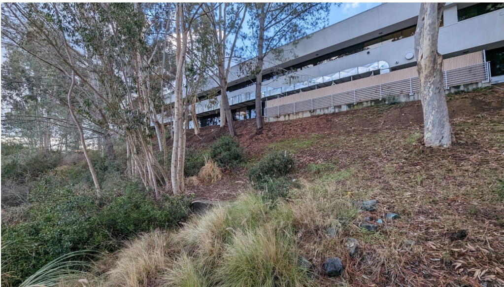
Overview of structure within APE, view to the southwest.
