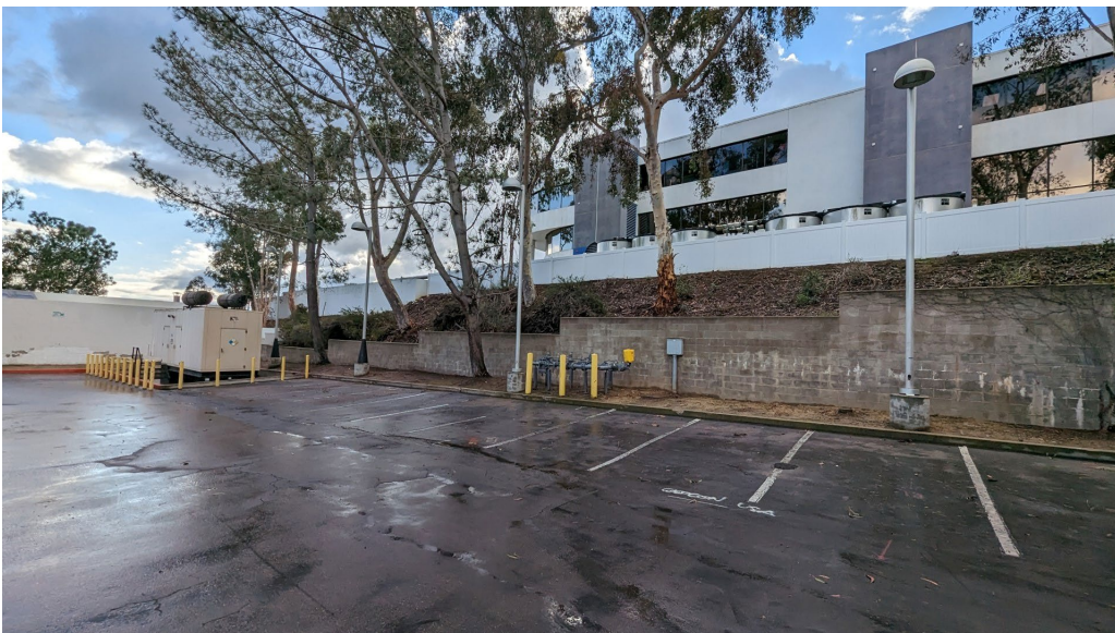
Overview of southern boundary of APE showing large cut in natural slope; view to the south.
