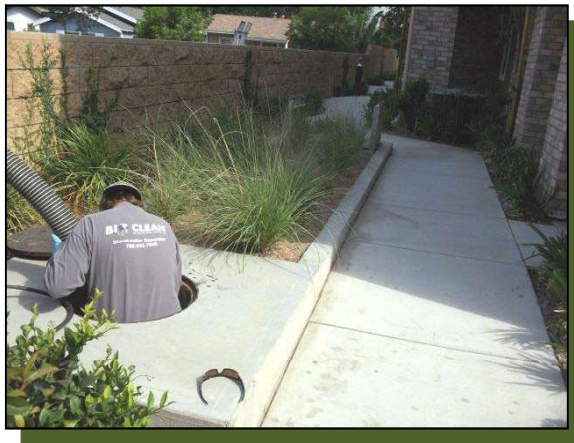
Vacuuming out of media filters.
