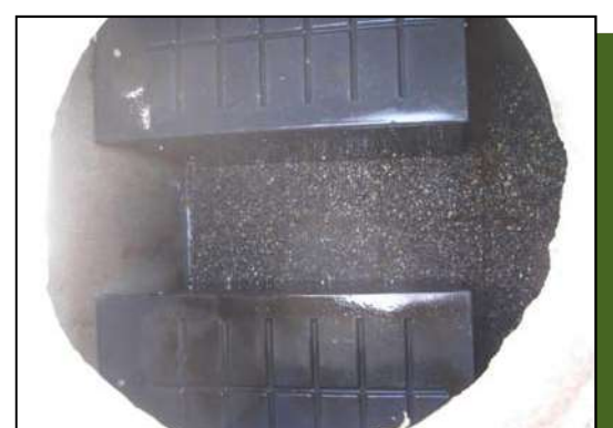
Fully cleaned separation chamber.
