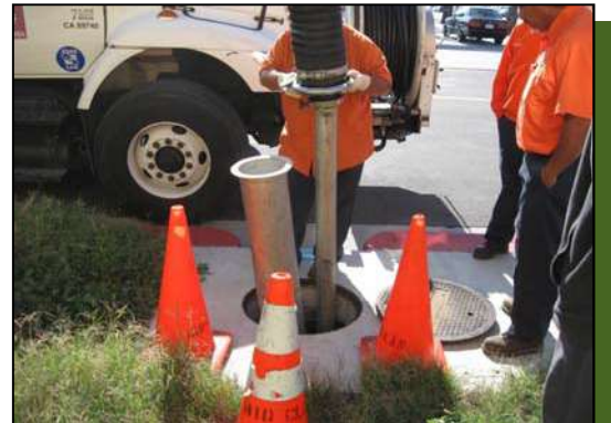
Insertion of vacuum hose into separation chamber.
