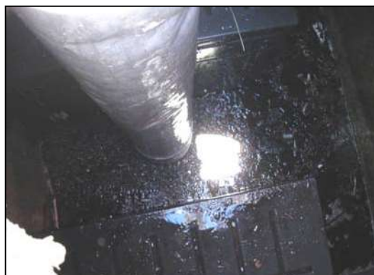
Removal of trash, sediment and debris.
