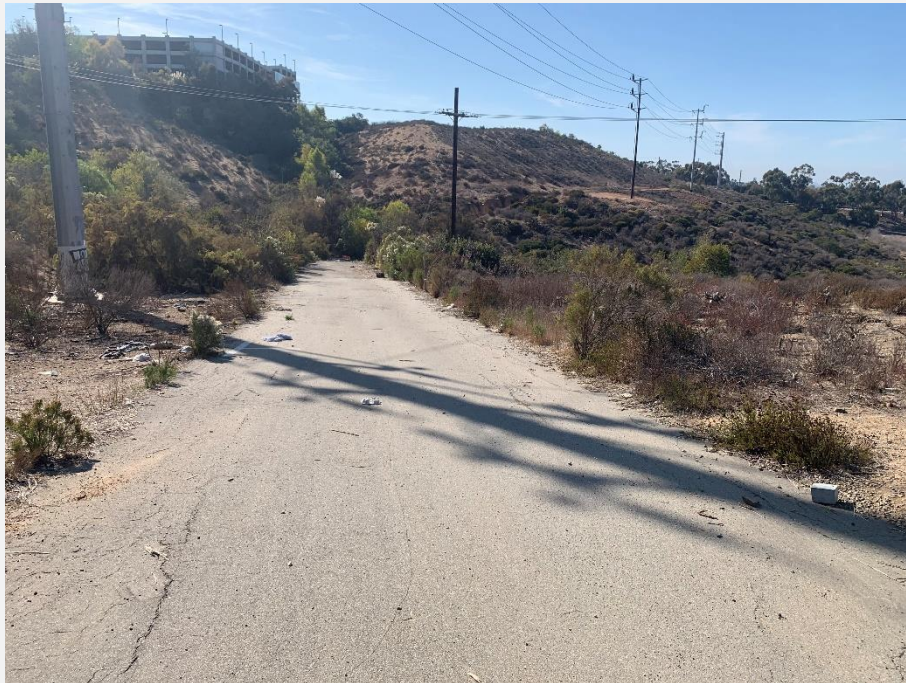
Photograph 4: Photograph looking west/southwest along the existing access road along the southern portion of the Project site. Photograph taken standing in the southeast corner of the Project site, at the proposed entrance to the development off Dennery Road.
