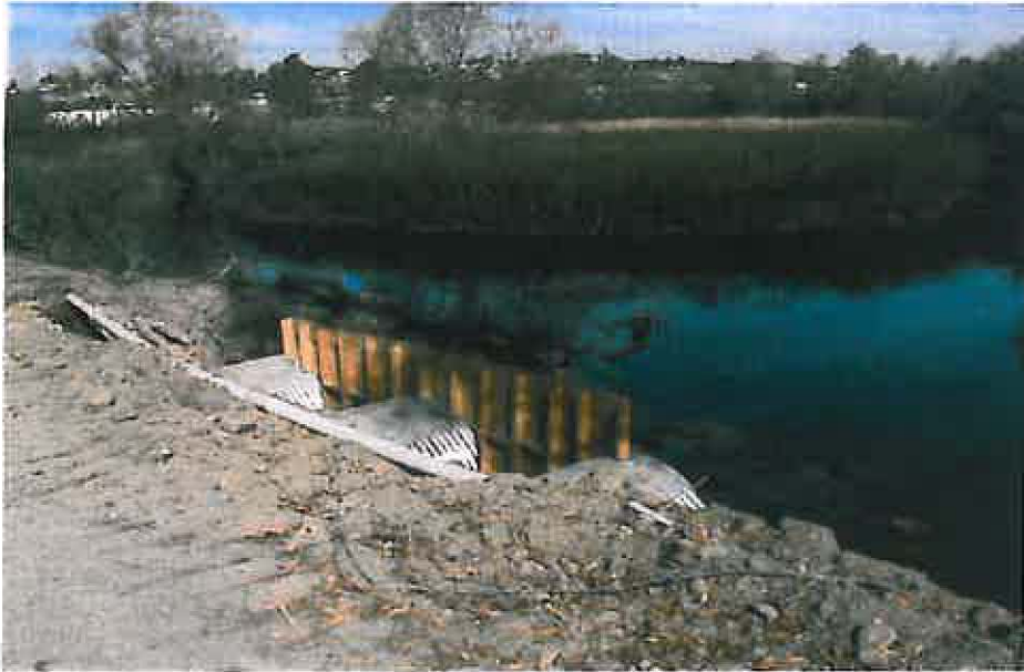
9. Otay River and bridge on the northern portion of the Property.
