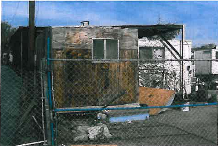
3. One of several residential structures on the Property.
