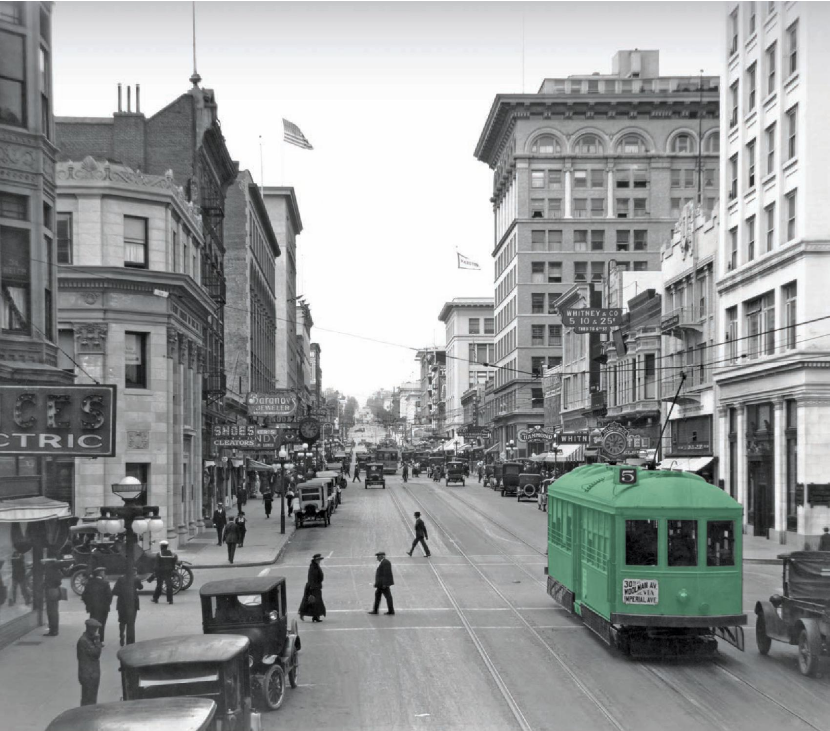
Looking north from E Street on 5th Avenue (1923) Courtesy of San Diego History Center
