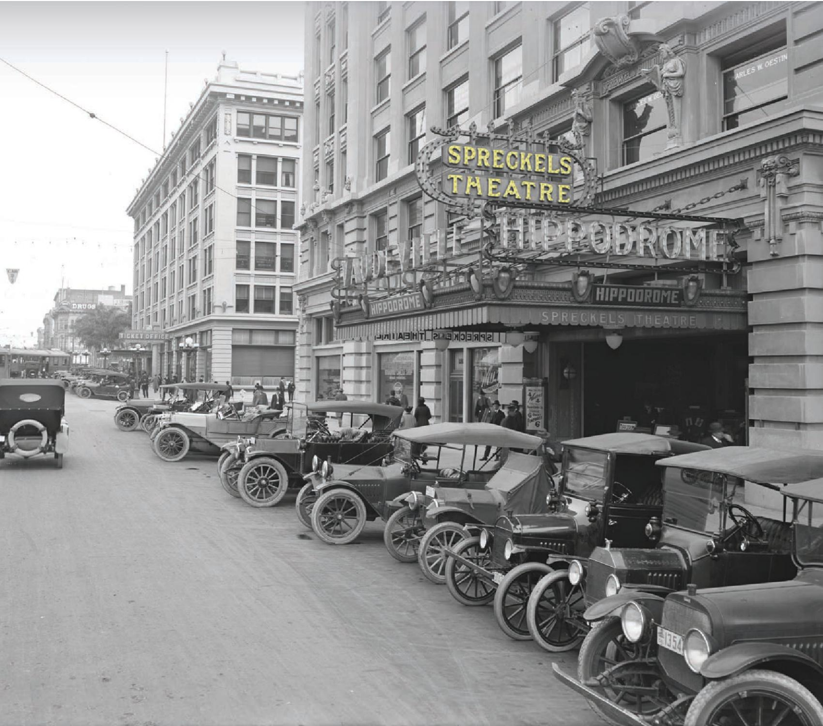
Spreckels Theatre, Broadway between 1st & 2nd Avenue (1918) Courtesy of San Diego History Center
