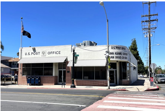
Figure 118: John Adams Post Office (ca. 1956) at 3280 Adams Avenue in the Mid-Century Modern style, appears to be the only extant post office dating to the 1900-1984 period in Mid-City.
