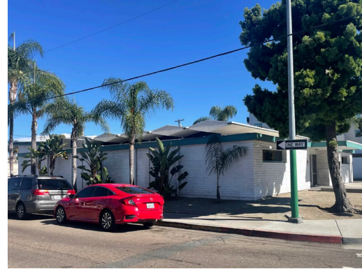
Figure 121: Former East San Diego Branch Library (4089 Fairmount Avenue), built in 1965 in the Mid-Century Modern style has a unique diamond-profile clerestory roof.
