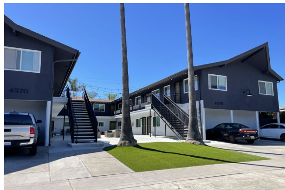
Figure 107: Apartment building (4570 Wilson Avenue, built c.1953-64) with a projecting peaked roof and tuck-under parking.
