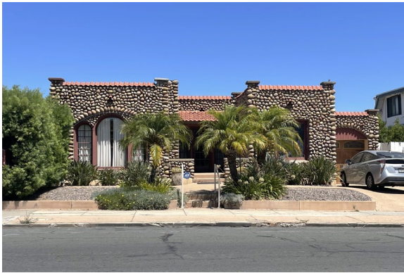
Figure 43: The Sharpless Residence at 3920 Adams Avenue (1927), utilizing the unique "pebble stone" façade treatment found in the area.
