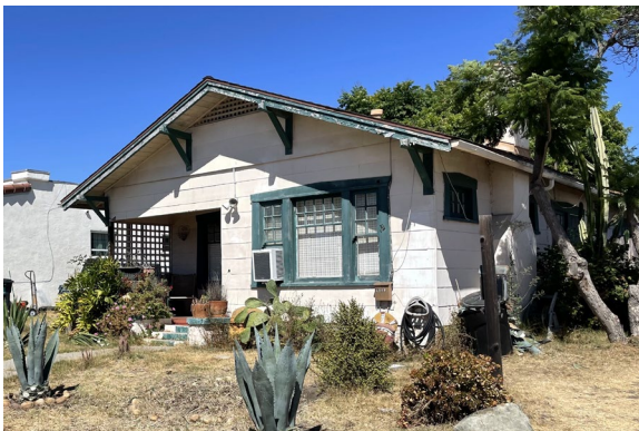
Figure 18: Circa 1900 residence within Normal Heights at 4869 Felton Street, cladding replaced, but original windows retained.
