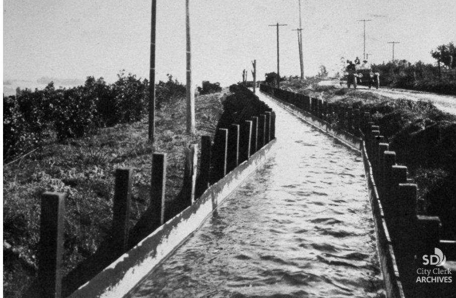
Figure 4: An example of the open flume at an unknown location in 1905 as built by the San Diego Flume Company. Since demolished. Source: San Diego City Clerk Archives.
