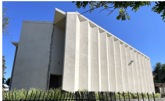
Figure 125: Church of Jesus Christ of Latter-day Saints (5299 Trojan Ave, 1962), designed in the Mid-Century Modern style by Deems & Martin.
