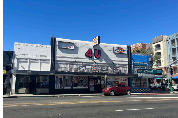
Figure 28: Streamline Moderne commercial building at 4292 University Avenue, built c. 1937.
