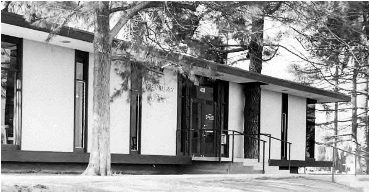
Figure 111: Remodeled Normal Heights-Kensington Branch Library (4121 Adams Avenue), 1963. Source: San Diego Public Library Special Collections.
