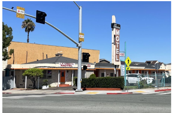
Figure 67: La Cresta Motor Court (4980 El Cajon Boulevard), built in the 1930s in the Minimal Traditional style, has a post-World War II neon sign and some alterations to material features.
