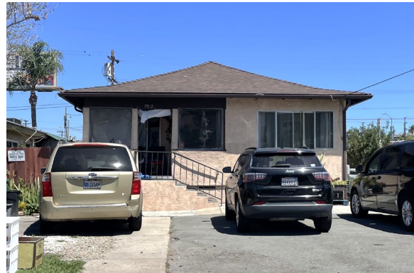
Figure 17: Circa 1900 residence within La Mesa Colony at 7012 Amherst Street, with rear addition.
