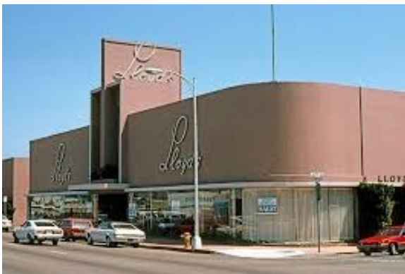
Figure 75: Lloyd's (4275 El Cajon Blvd, built 1948) chain furniture store with streamline elements and large signage to attract passing automobiles. Source: Vintage San Diego, Facebook.
