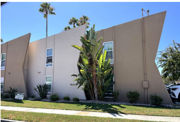
Figure 106: Mid-Century Modern apartment building (6271 Madeline Street, built 1963) with a unique staggered façade profile.
