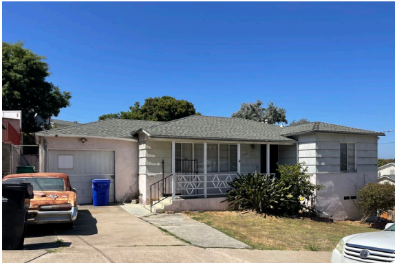
Figure 98: Typical Postwar Minimal style house built in the early 1950s in Westwood Hills, large tract developed by O.D. Arnold and Sons.
