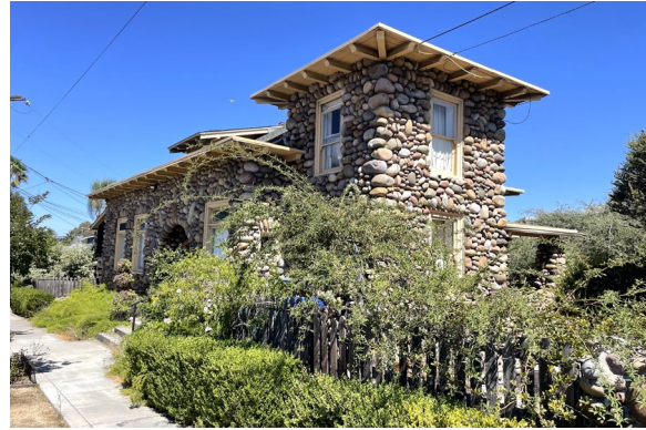
Figure 15: The Brenkert House at 3805 Merivale Avenue (1912) in the Bonnie Brae neighborhood of Normal Heights, with the unique “pebble stone” façade treatment.
