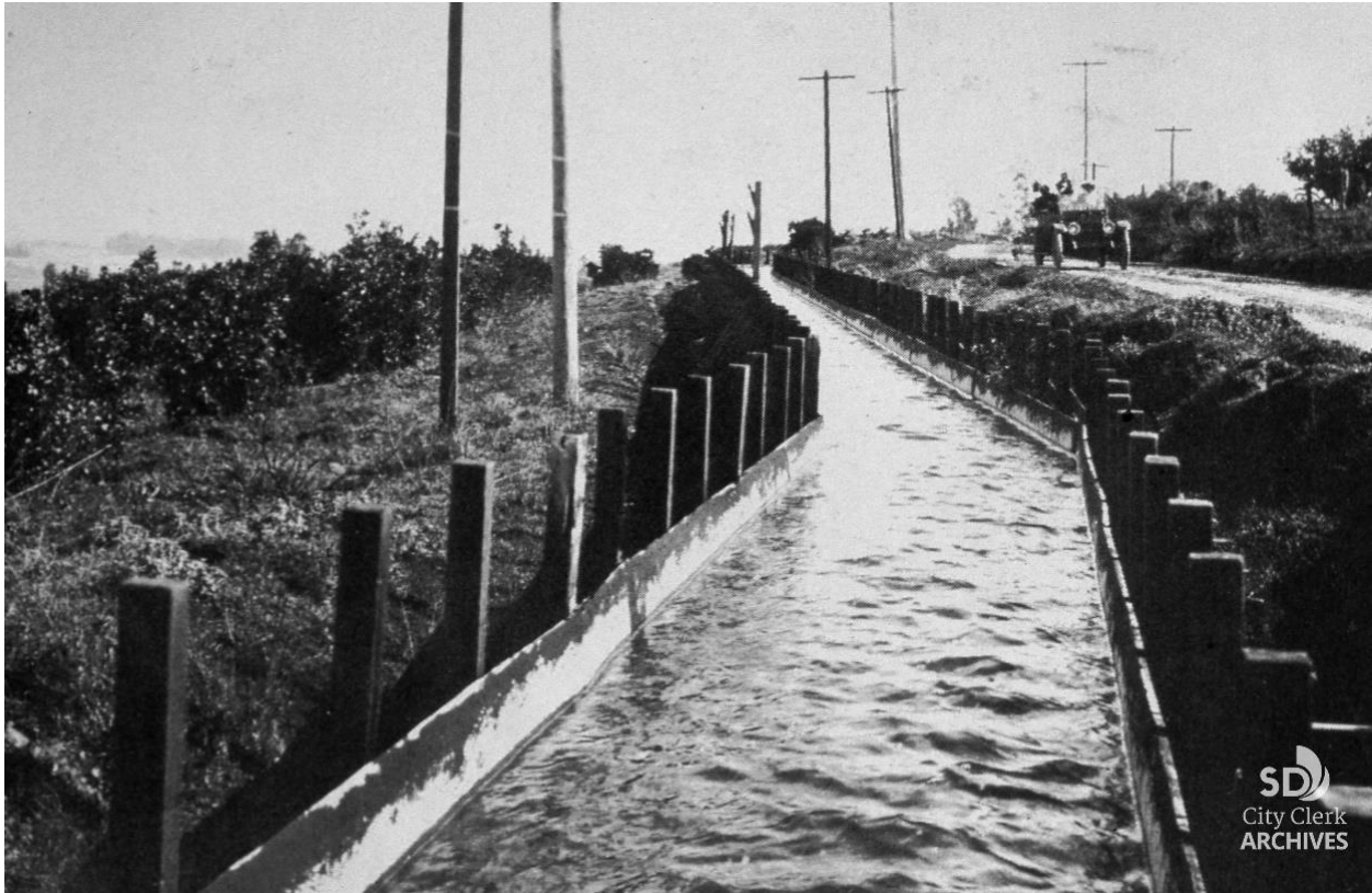
Figure 4: An example of the open flume at an unknown location in 1905 as built by the San Diego Flume Company. Image Source: San Diego City Clerk's Office.
