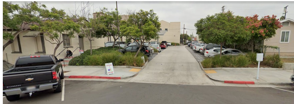
C. EXISTING ALLEY WAY FROM NEWTON AVE. W
