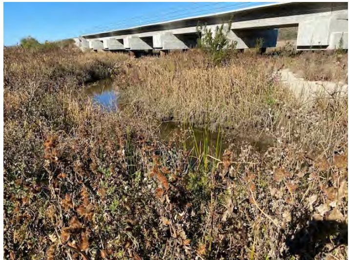
Significant Dry Weather Flows – Existing Channel - Lower Downstream Trestle
