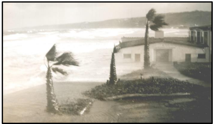
Plate 3.2–4: The Marine Room during a storm in 1944. (Photograph courtesy of the Marine Room)
