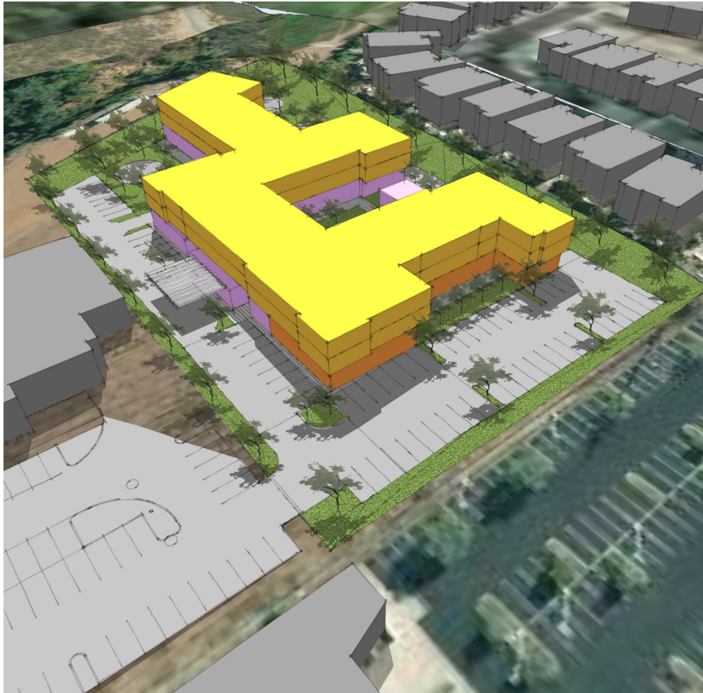
Aerial View from Northwest
