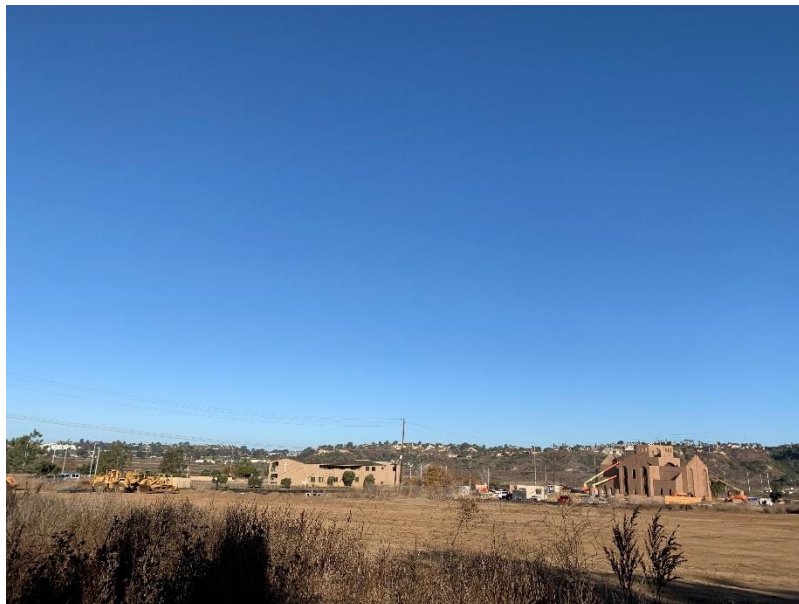
Photograph 23. Looking northwest across the subject property to the active construction site to the north and the Harvest Evangelical Church to the west.
