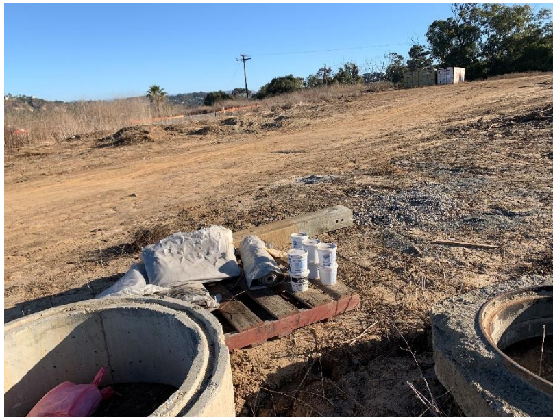
Photograph 19. Construction materials store on the subject property.
