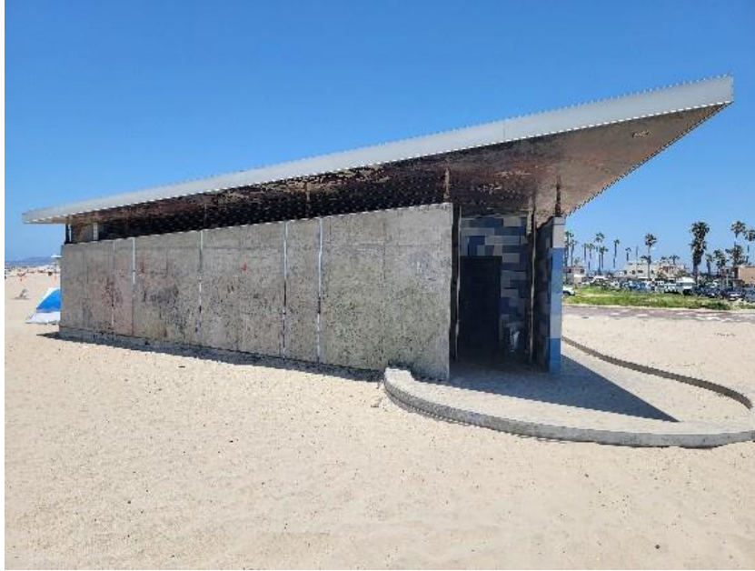
Photograph 3: Ocean Beach – Dog Beach. Modern bathroom facility.
