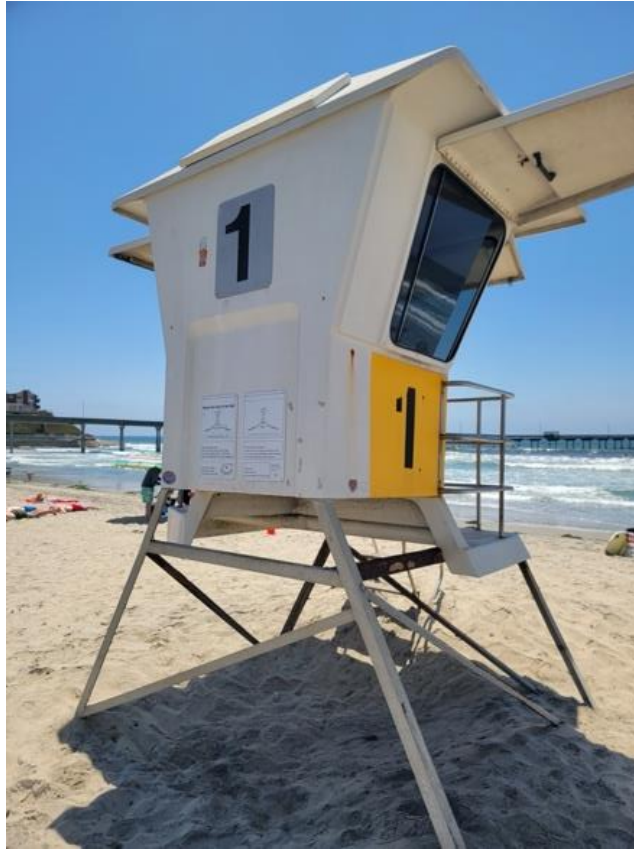
Photograph 15: Ocean Beach – Pier. Modern fiberglass and metal pole lifeguard tower.
