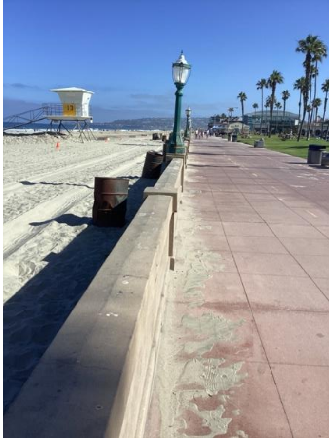
Photograph 13: Mission Beach. Beach and boardwalk survey area.
