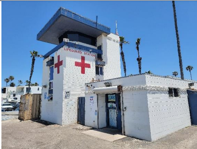
Photograph 16: Ocean Beach – Pier. Modern lifeguard station constructed in 1980 & 1981.
