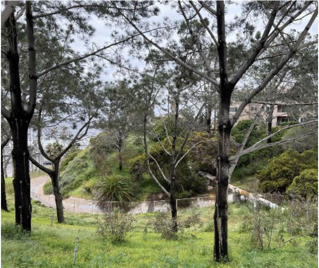
Figure 5.3-5. Concrete Channel Adjacent to the North of the Pacific Beach – Tourmaline Surf Park Project Site
