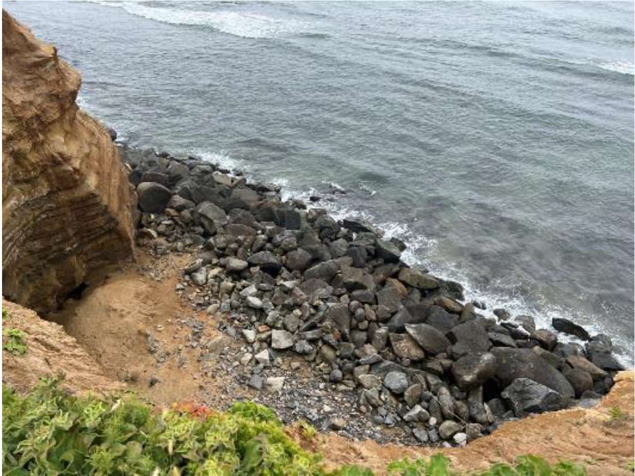
Figure 5.5-4. Rock Riprap at the Bottom of Sunset Cliffs
