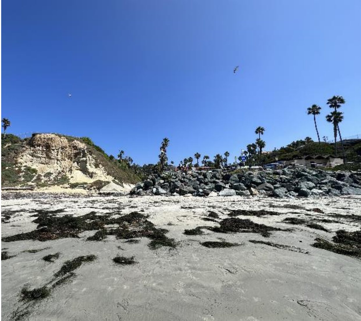
Figure 5.5-3. Cobble Berm and Riprap and Winter Sand Berm on the Pacific Beach – Tourmaline Surf Park Project Site
