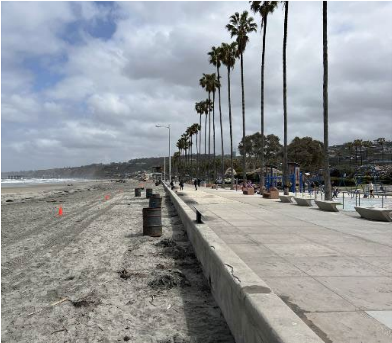
Figure 5.3-9. Paved (Developed) Pedestrian Pathway (La Vereda) on the La Jolla Shores Project Site
