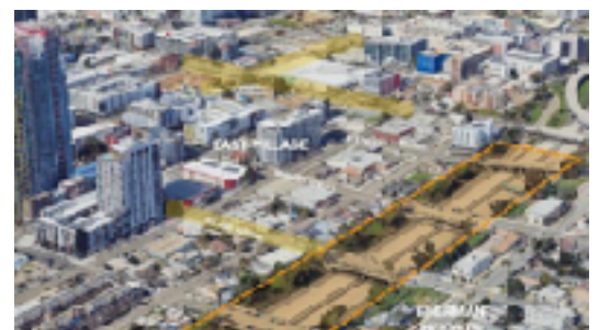
I-5 lid locations: top, 6th Ave.-Park Blvd., bottom, G-J streets, San Diego Commons and Urban Division Story Map, 2023
