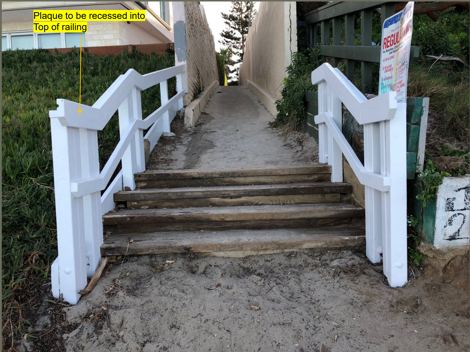
Plaque Location 5 – Winamar Stairs
