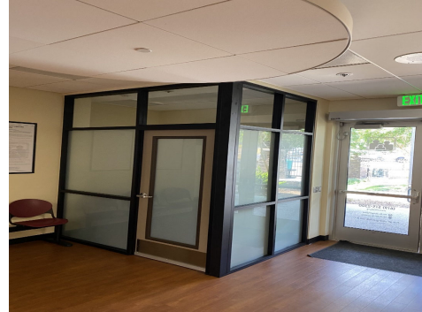
Family Health Centers of San Diego Diamond Neighborhoods Remodel
