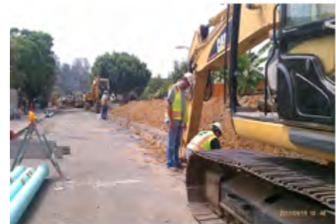
TCDB installs deep sewer mains in a residential neighborhood.
