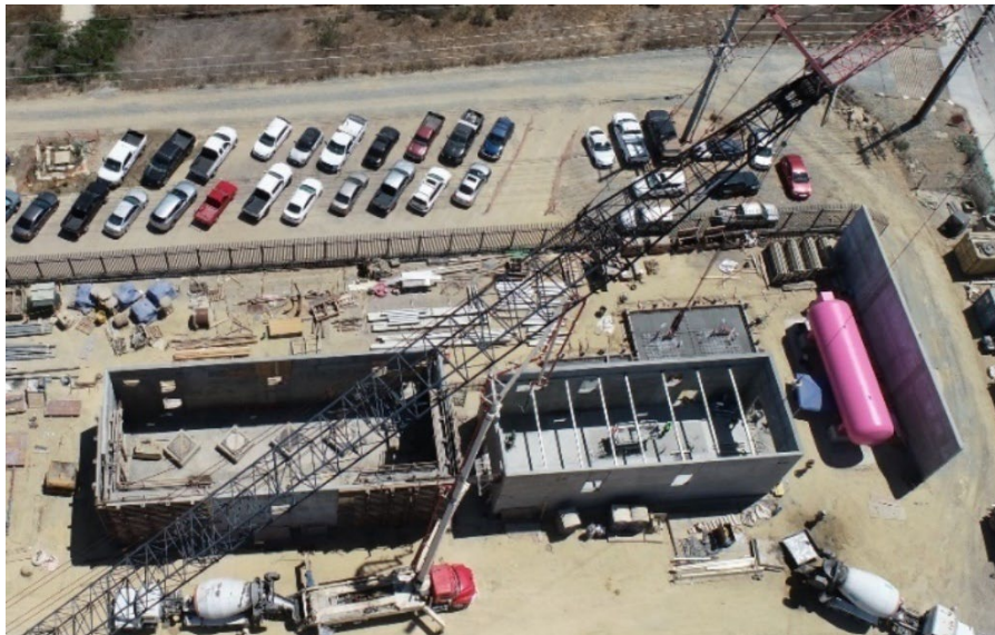
North City Pure Pump Station
