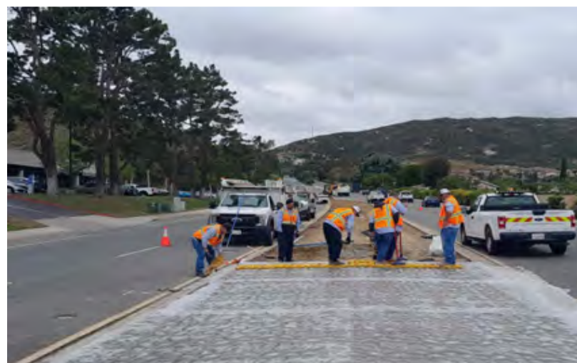
City crews constructing a center median.
