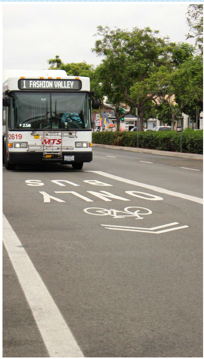
Flexible (flex) lane along El Cajon Boulevard
